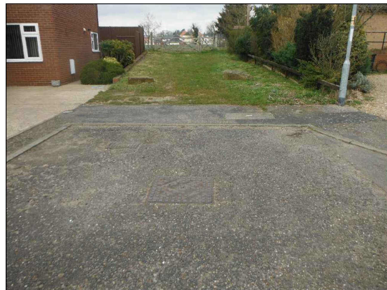
From Sandstone Way looking up existing access to site. Please note manhole covers in road for connection purposes.
