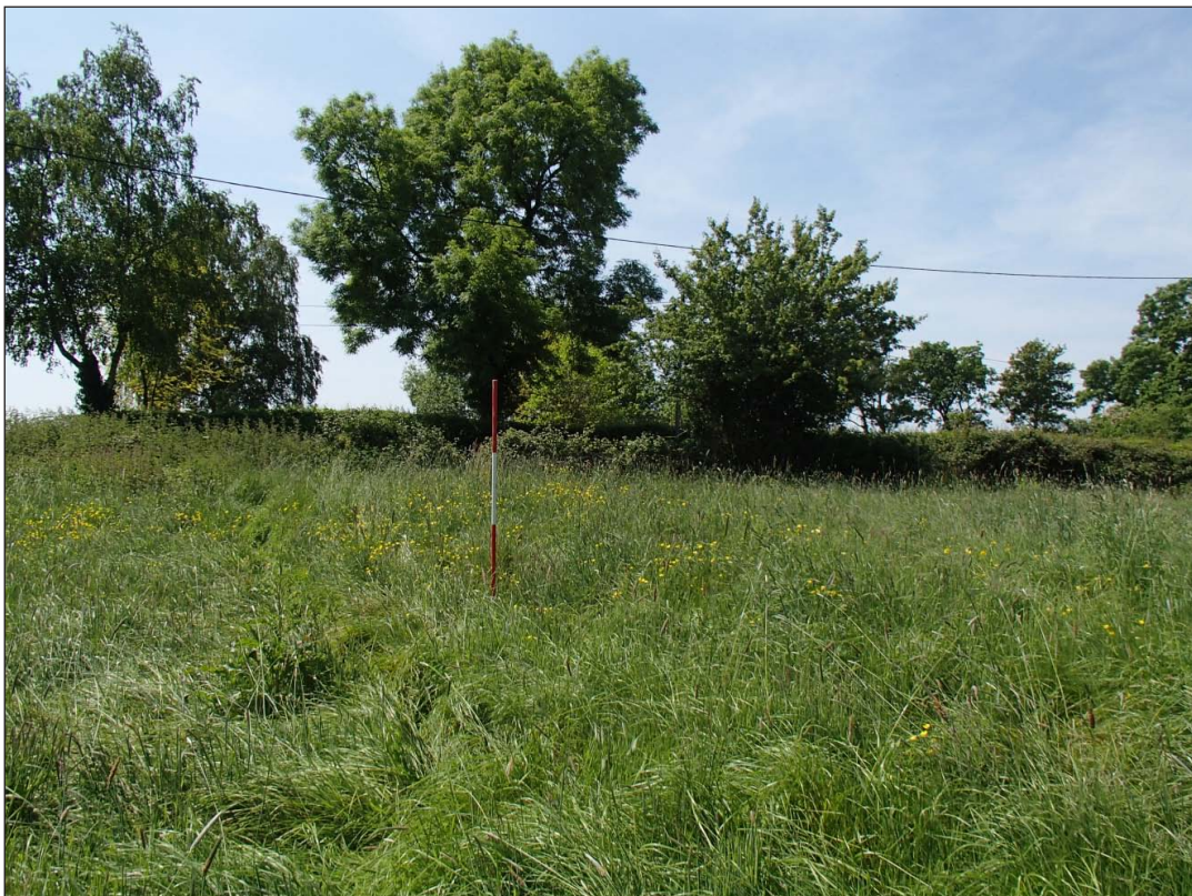
Fig. 10 - Monument 2B, west side of embankment
