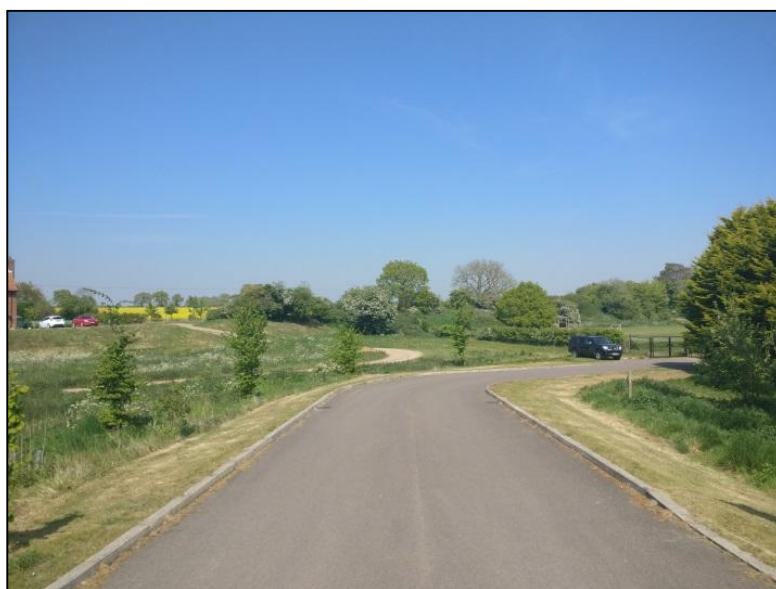
Figure 4-2 Hempnall Primary School Access Road
