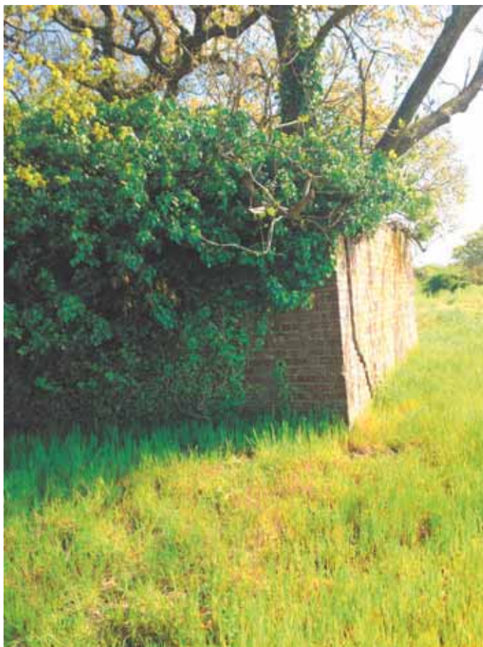
Plate 23: WWII military structure immediately south of the northern boundary line
