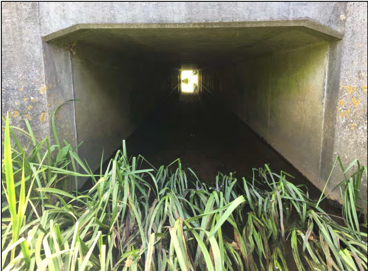
Figure 21: Concrete rectangular culvert under A140
