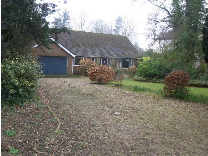
Figure 10. The western access corridor.
