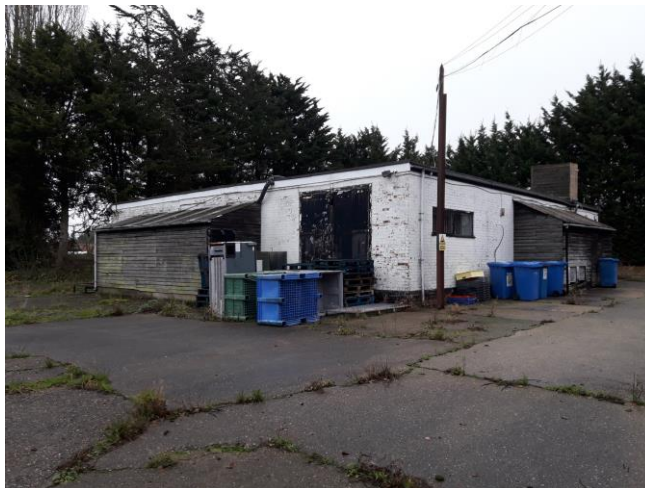
Photograph 2 The Office Building. Viewed from the north-east looking south-west
