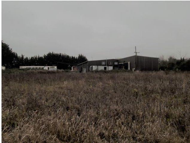
Photograph 1 Former Meat Processing Factory, Building B1. View from the north looking south.
