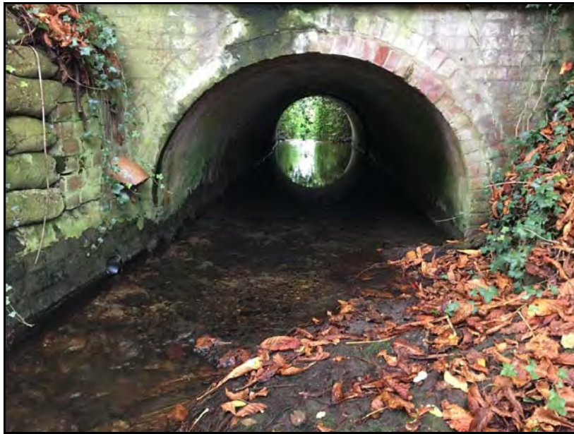
Figure 19: Photo of brick arch bridge entrance (Source: BB Surveys)
