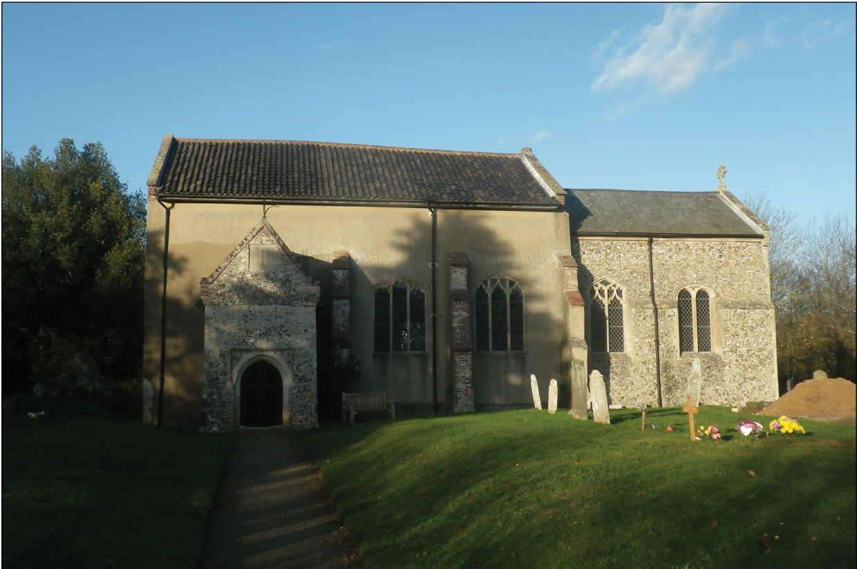
Plate 1: St Peter's Church, Easton (viewed from the south)
