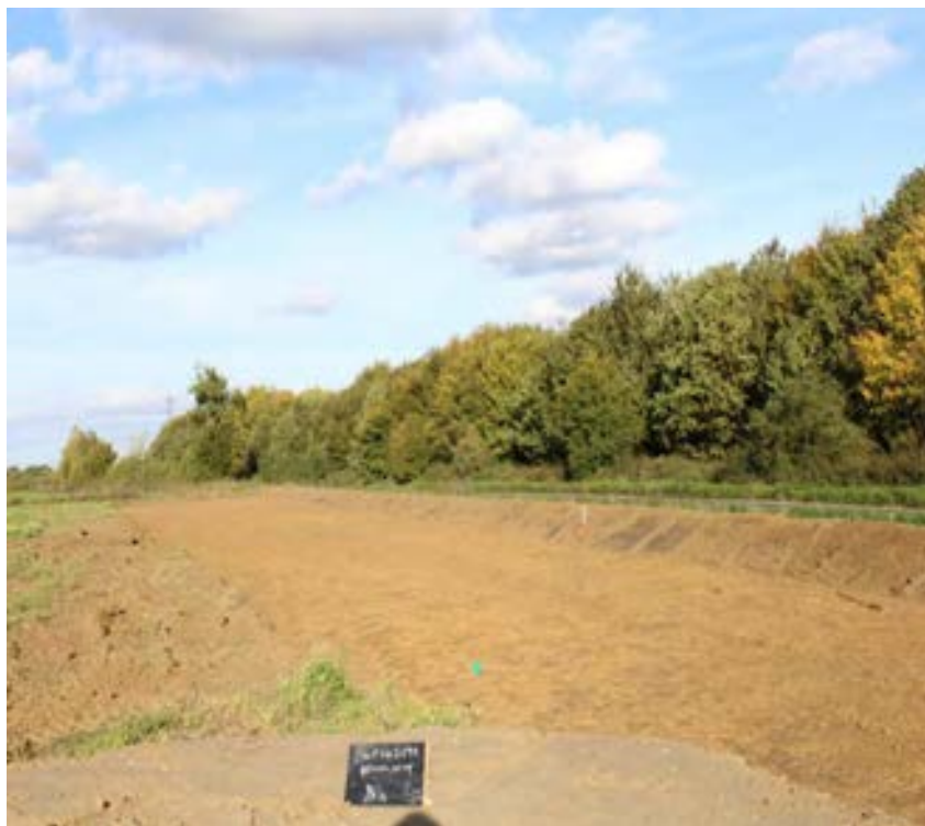
Plate 1: Easement strip on west side of Colney Lane, facing north-east
