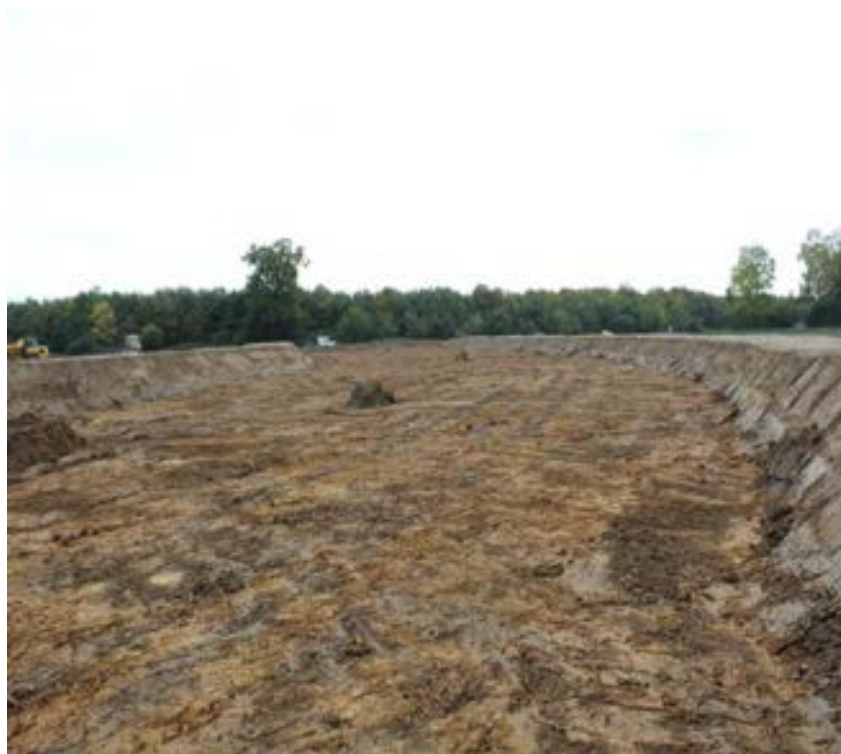
Plate 3: South-east end of strip, facing south-east
