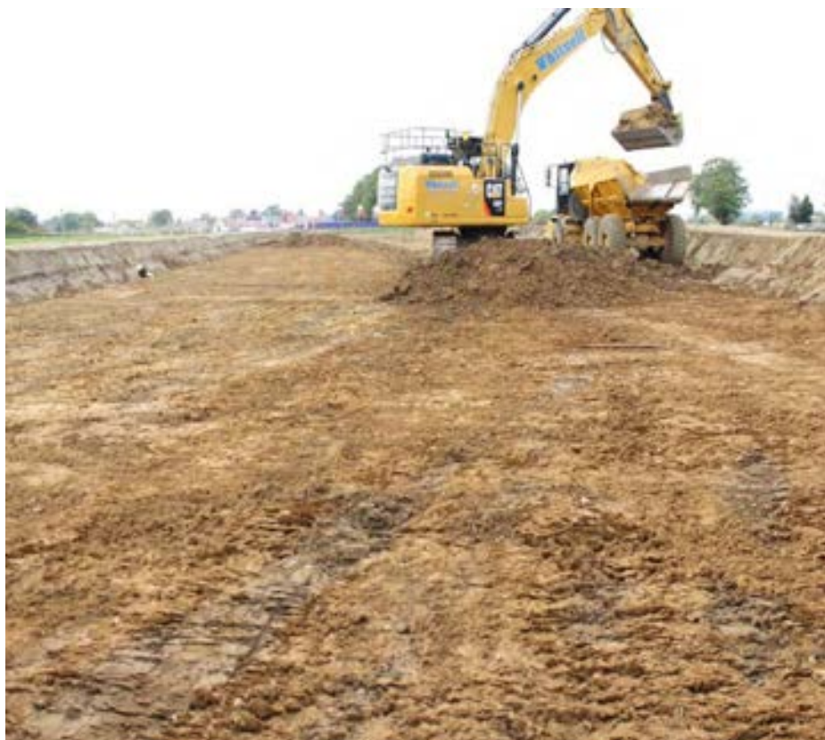
Plate 5: Working method of road strip, facing north-west
