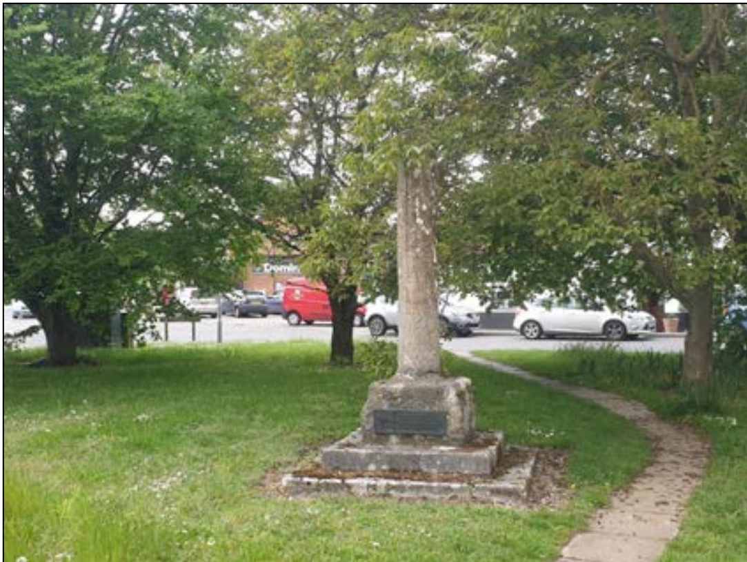
DP 48. View towards the proposed development site incorporating the Grade II listed and Scheduled Monument of the Market Cross, Drayton
