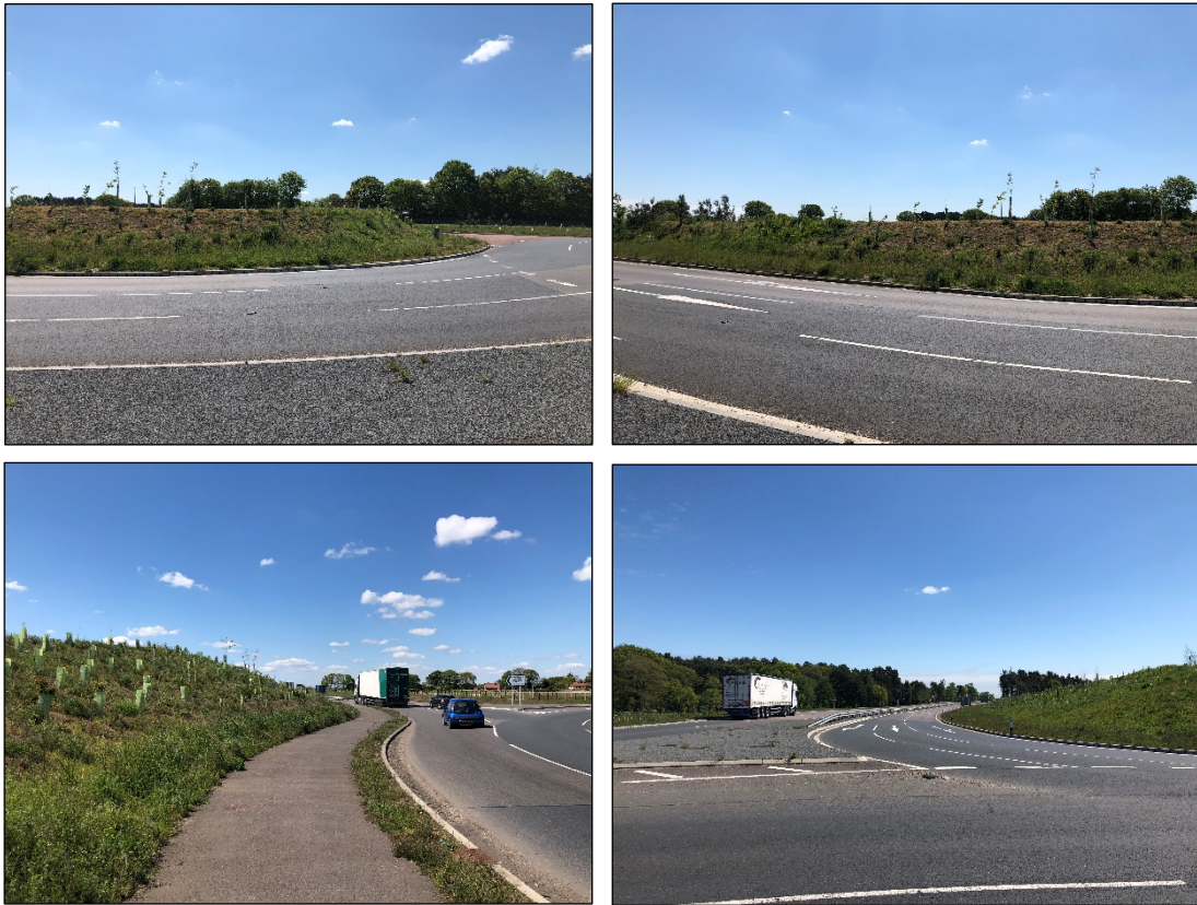
Figure 7.4: Photographs Showing Existing Earth Bunds
