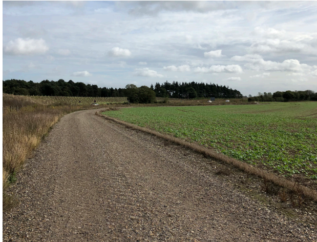
Northern edge of site with adjacent 'bund' and farm access route
