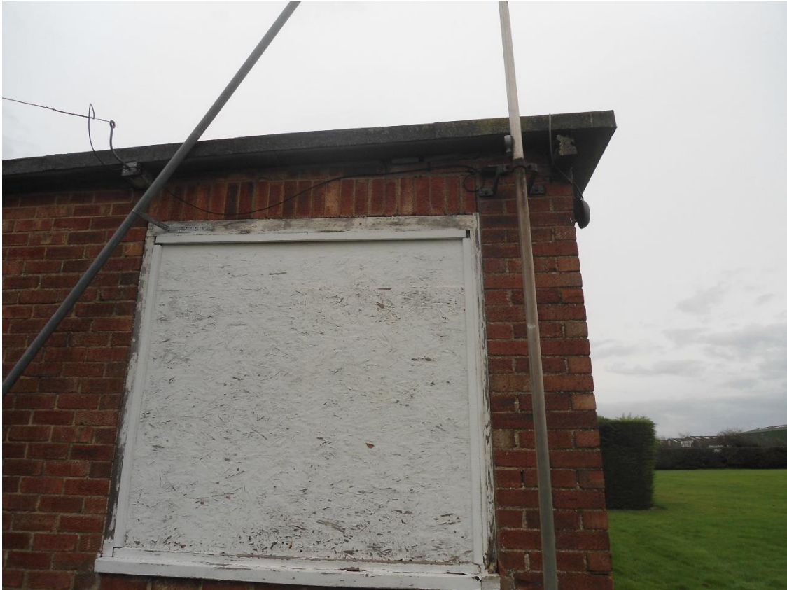
Photo 9: Side wall of site showing roofing material
