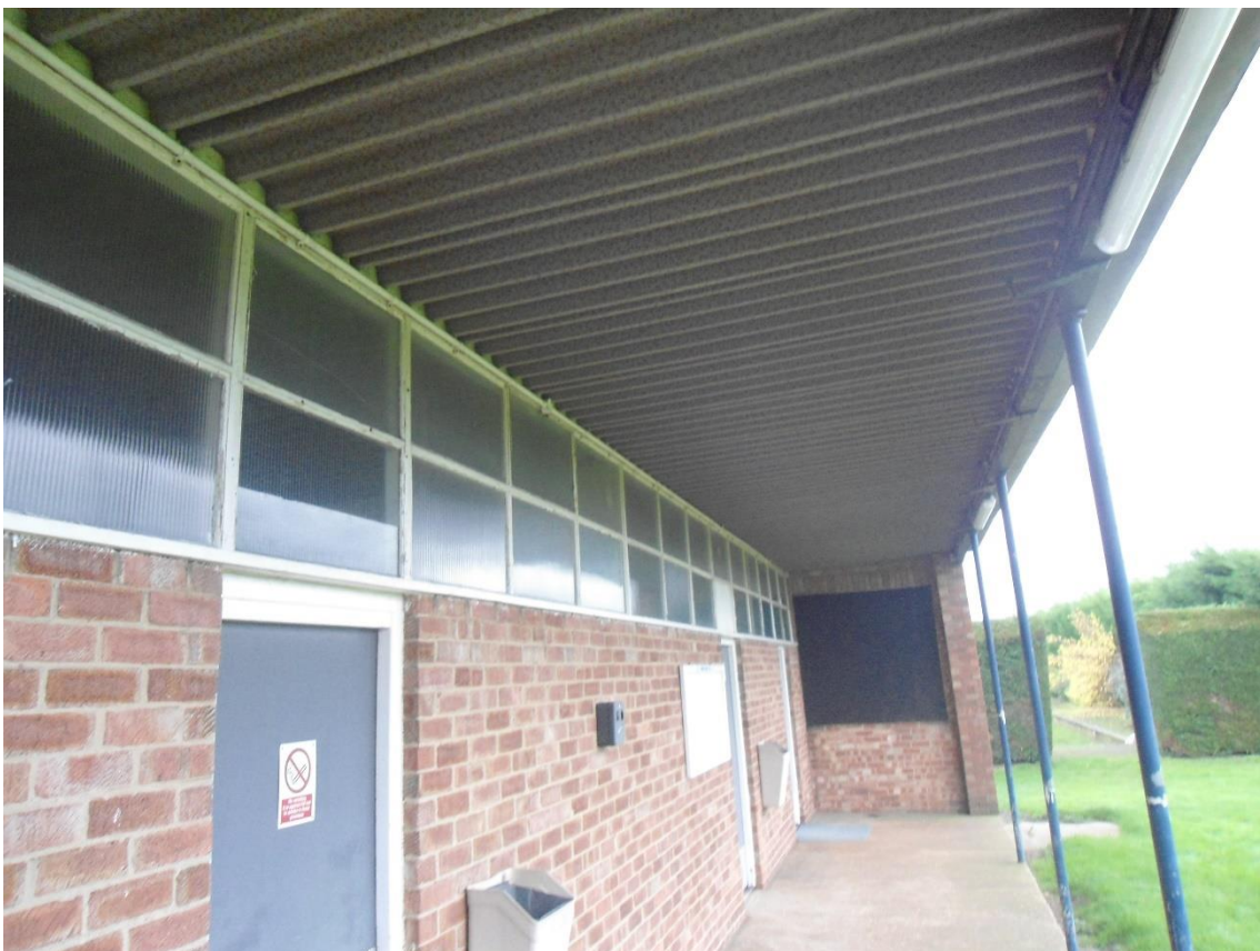
Photo 8: Front face of outbuilding
