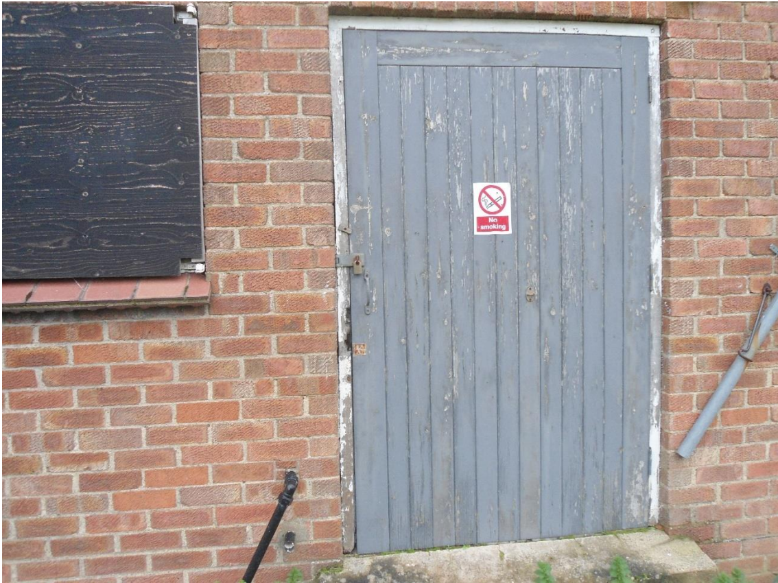
Photo 11: Side view of outbuilding showing sealed doors and windows
