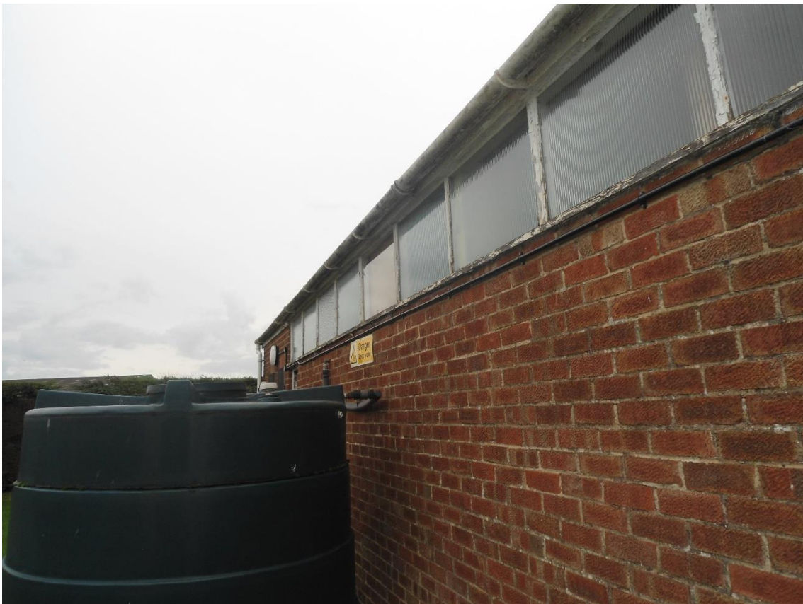
Photo 12: Side of outbuildings showing sealed windows
