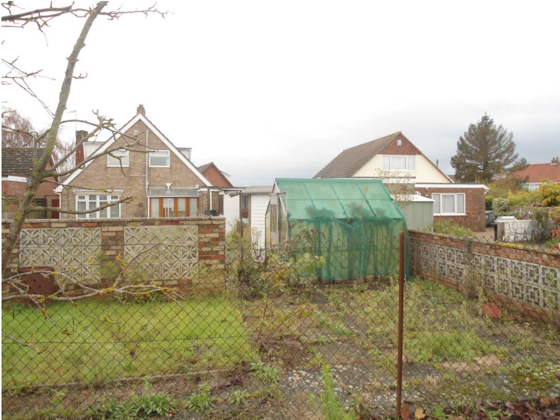
Photo 19: Property on western edge of site
