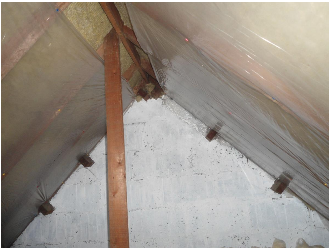
Photo 38: Further view of the roofspace at the gable end
