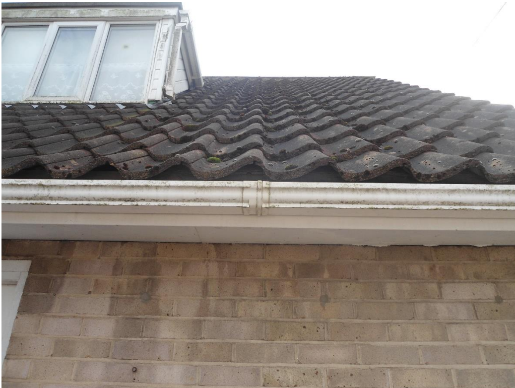
Photo 36: Concrete pantile roof with small spaces along the eaves
