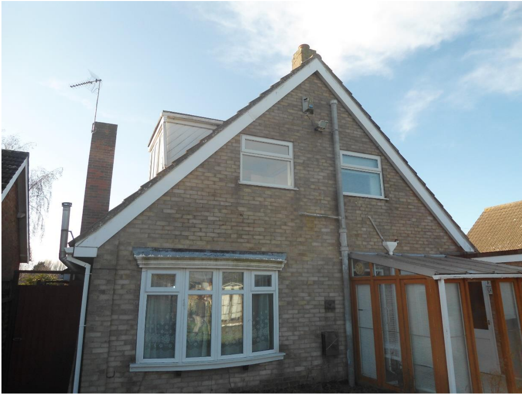
Photo 33: View of the eastern elevation
