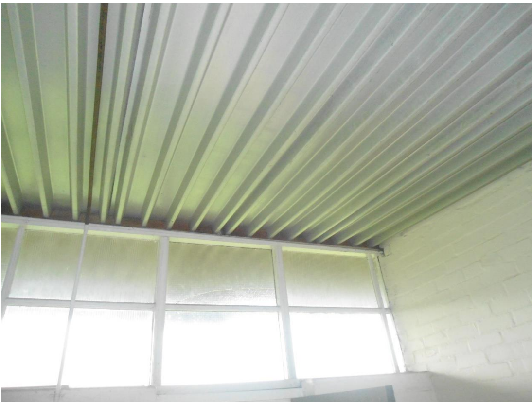
Photo 14: Corrugated roof on inside of building
