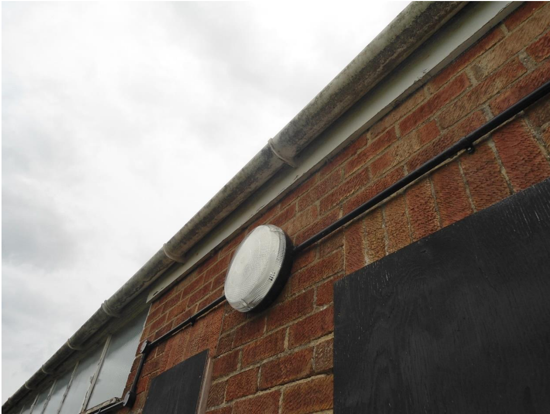
Photo 13: Fascia around side of building
