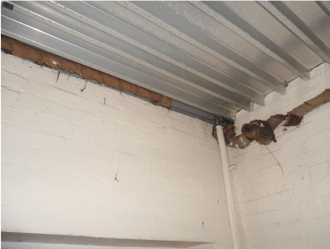
Photo 15: Well sealed roof on building with no bat access
