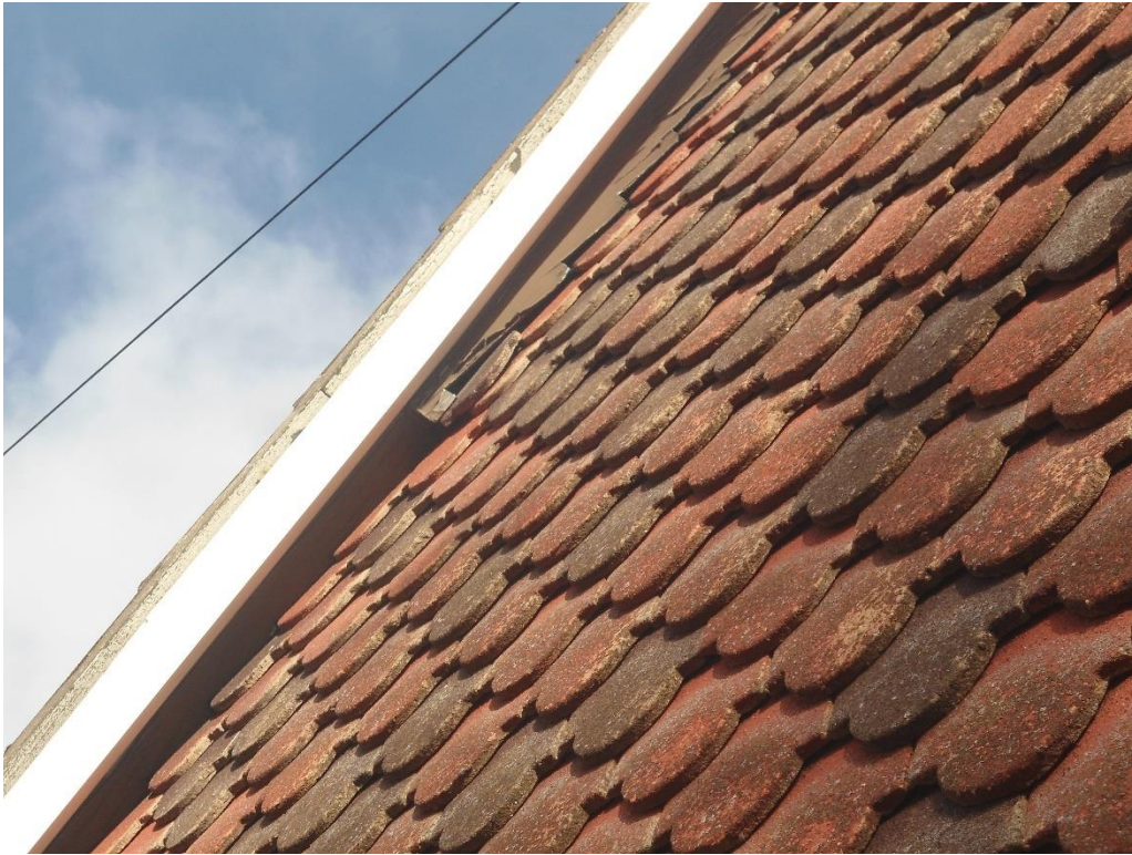
Photo 35: Further view of soffit cavities
