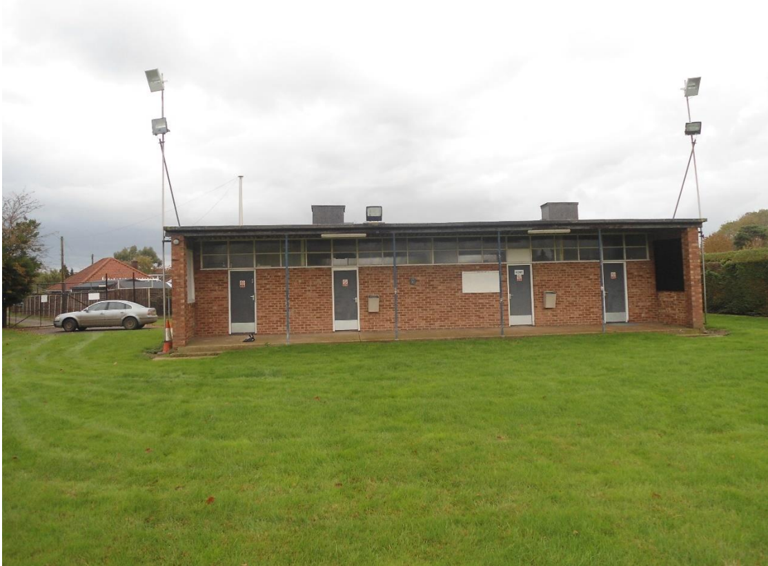
Photo 3: Outbuilding on site, formerly changing rooms
