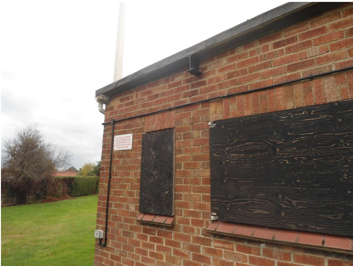
Photo 10: Side view of outbuilding showing sealed windows
