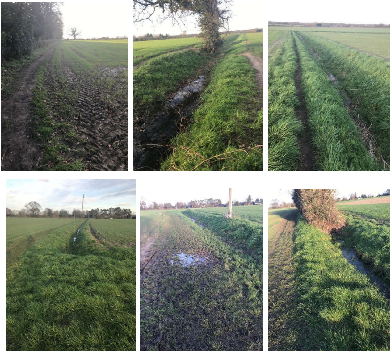
Figure 3.7 – Central and Southern Drainage Ditches (some ponding in flatter locations)
