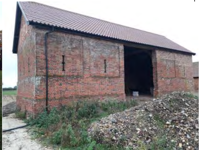
Photo 22: Building, Lower Park Farm, high bat potential.
