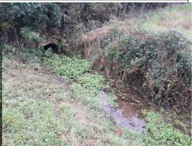
Photo 18: Watercourse crossing under the main farm track.
