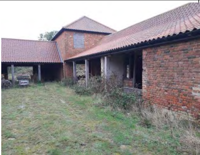
Photo 23: Building, Lower Park Farm, high bat potential.
