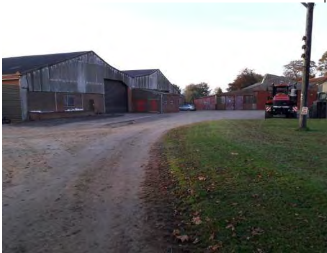
Photo 21: Buildings, Park Farm, Low bat potential
