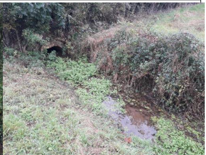
Photo 18: Watercourse crossing under the main farm track.
