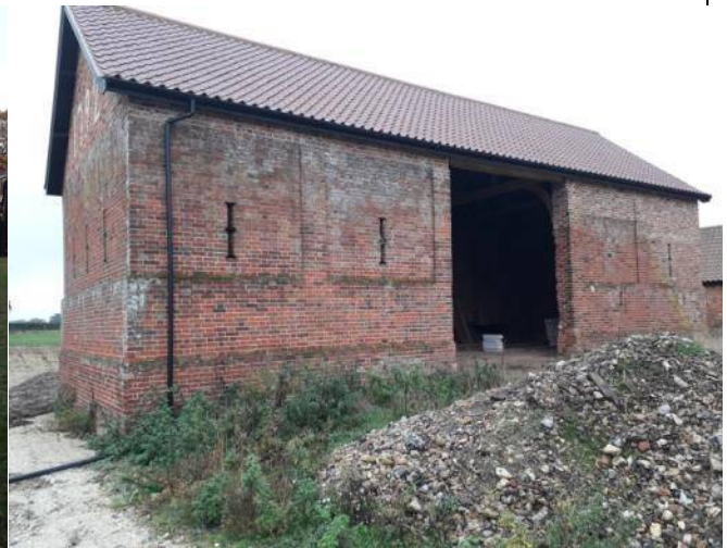
Photo 22: Building, Lower Park Farm, high bat potential.
