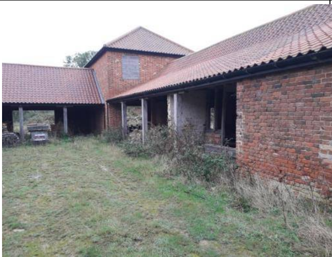
Photo 23: Building, Lower Park Farm, high bat potential.
