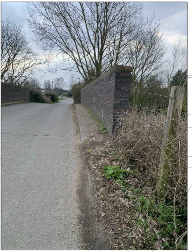
Narrow footpath over bridge
