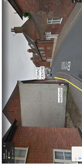
8. Narrow bends with severely restricted footpath on both sides, path is blocked by taller buildings requiring crossing with poor visibility around bends
