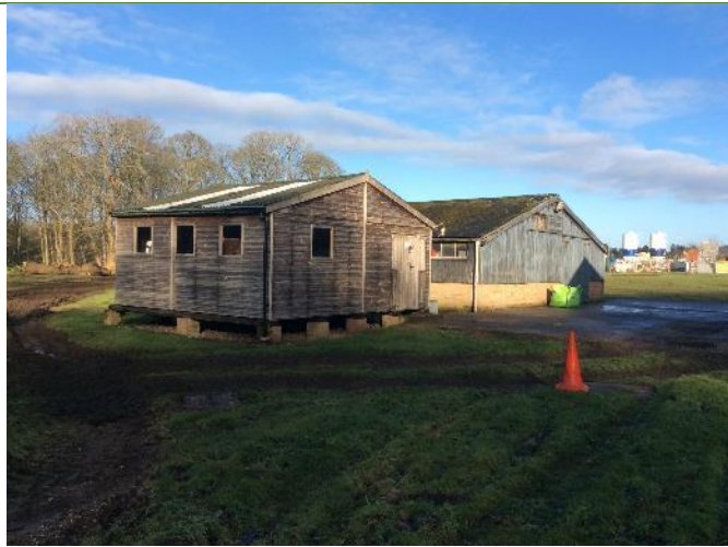
Photograph 7. Building B4 (elevated shed).
