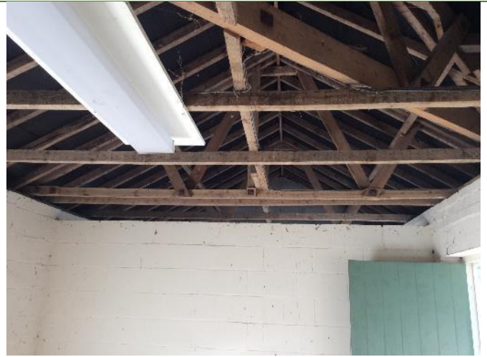
Photograph 4. Internal structure of stables.
