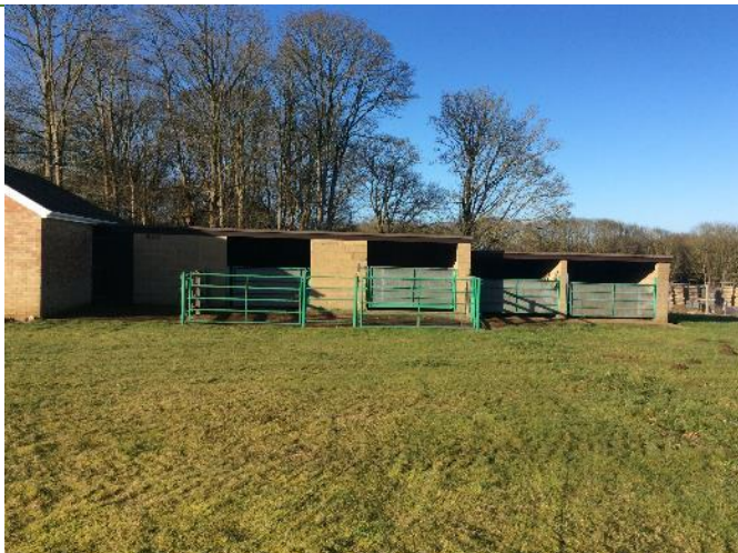
Photograph 5. Building B2 (older stables/animal sheds).
