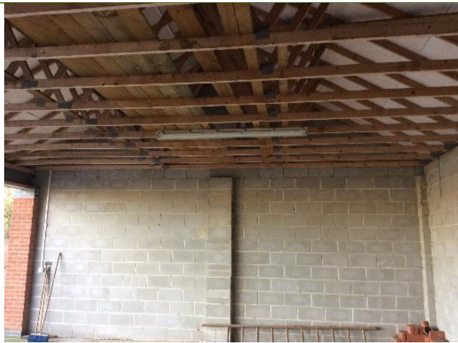
Photograph 9. Interior structure of Building B5.
