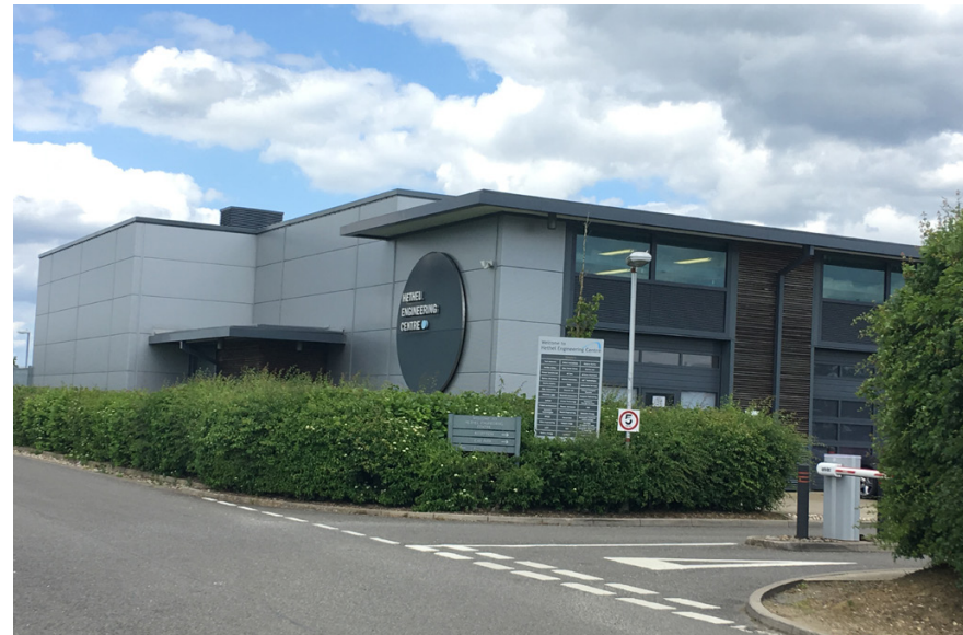
Viewpoint 9: Looking north west
