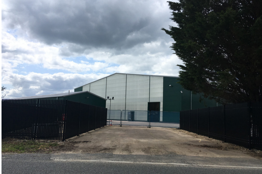
Viewpoint 8: Potash Lane, looking north west
