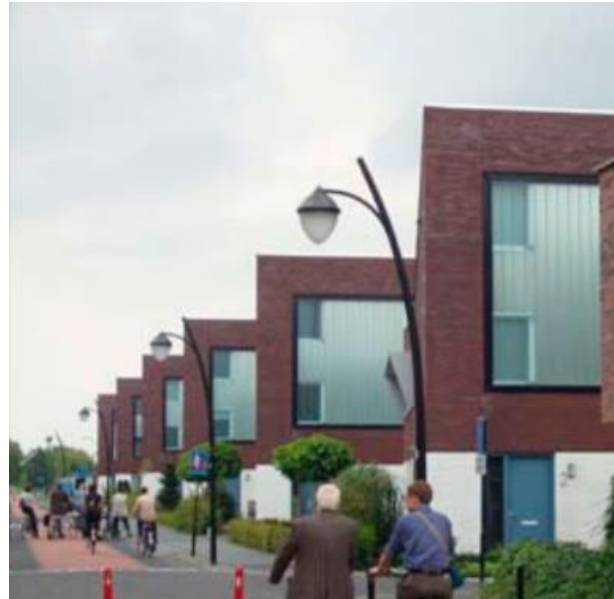
Amersfoort a small historic city in The Netherlands, with its three new suburbs: Kattenbroek, Nieuwland and Vathorst. Amersfoort hosts safe walking and cycle routes through the site reduce car dependency
